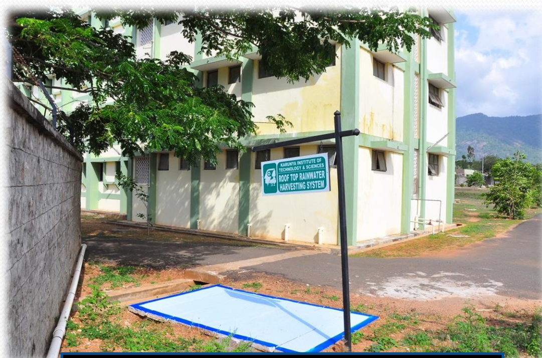
20. NEAR SUNDHARAJ RESIDENCE
