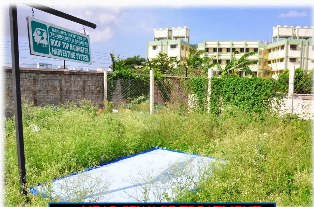
17. NEAR SEWAGE TREATMENT PLANT
